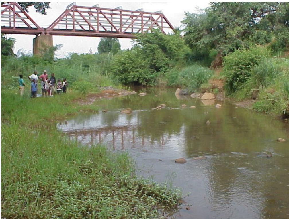
14. Letsitele tank – shallow pool downstream of bridge
